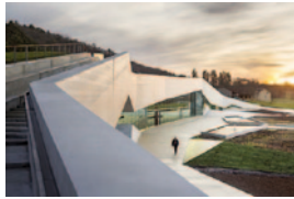
Snøhetta_Lascaux_BoeglyGrazia.jpg Lascaux IV – Centre International d’Art Parietal, Montignac (F) Credit: © Luc Boegly + Sergio Grazia
